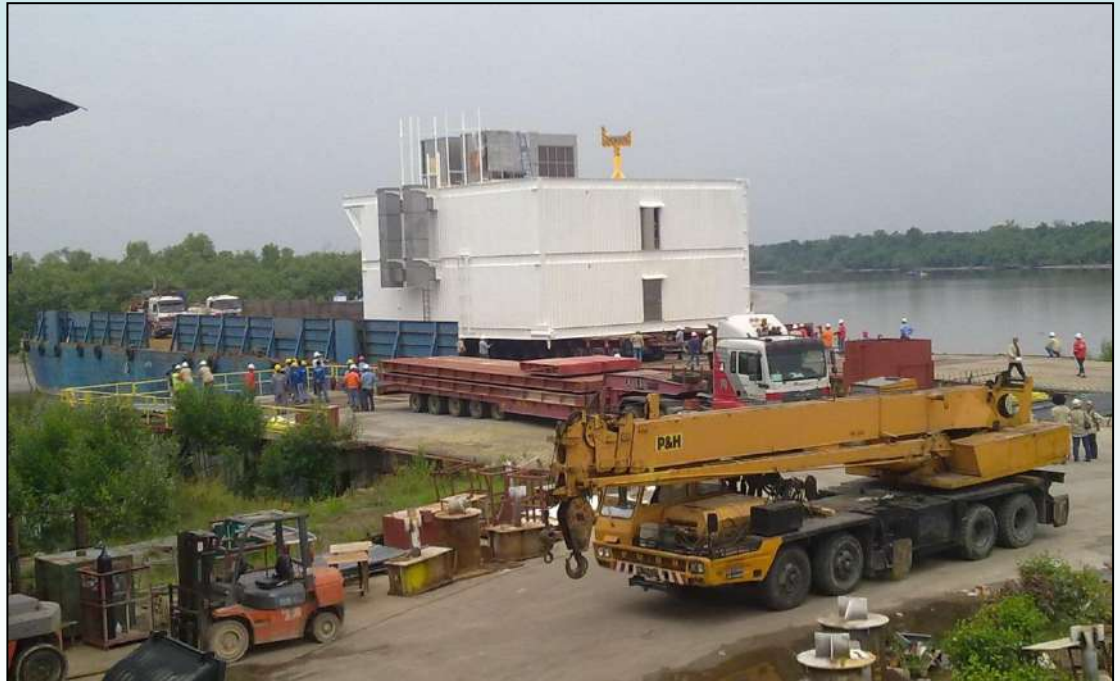
LQ Module 2 & 3 Load Out on 19 th Jan 2013
