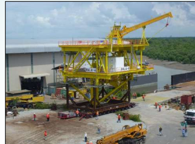
Balai platform load out
