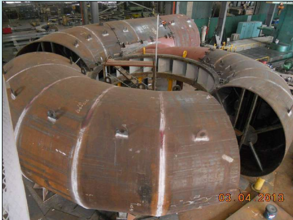
Spiral Case and Embedded Parts - Completed July 2013
