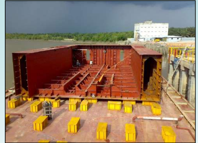
Hull Assemble on Floating Dock
