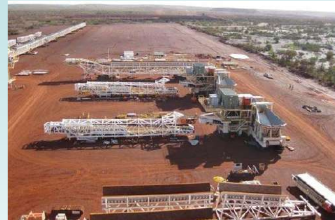
Bridge 45 & System #1 TTMSs
