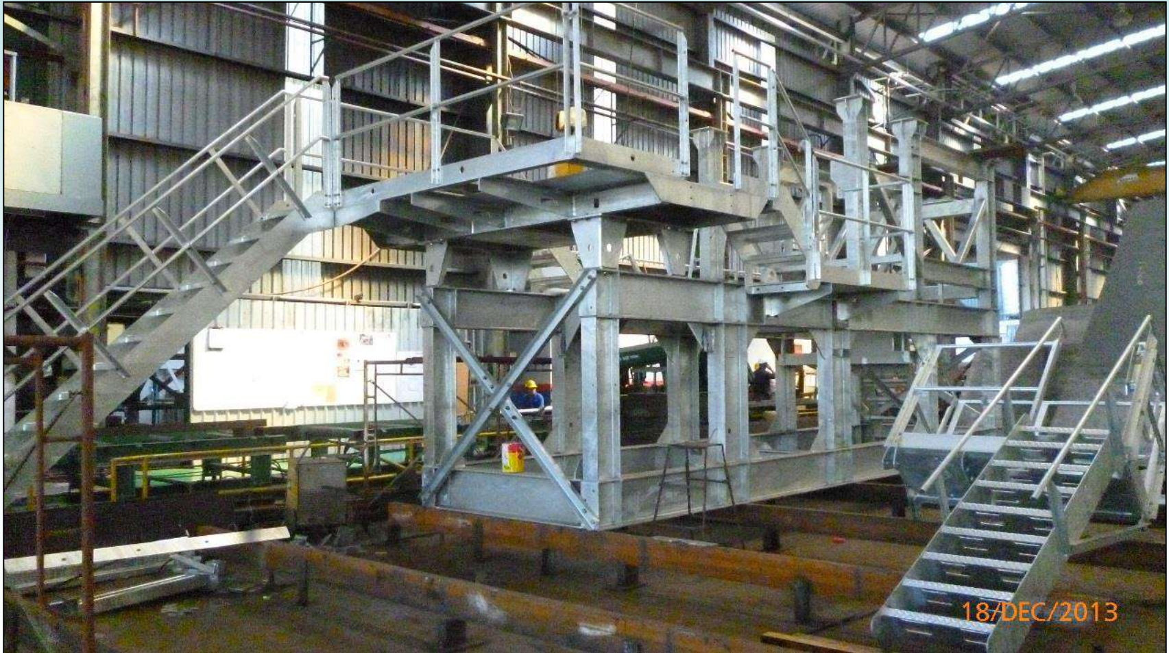
MJ 42A Base Structure
