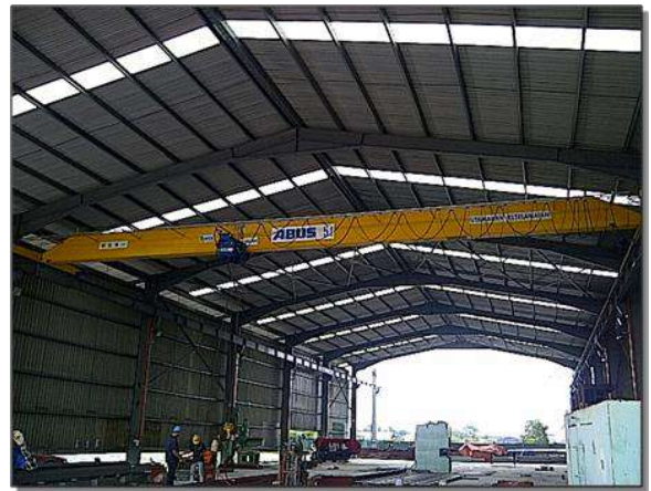
OVERHEAD CRANE 5 ~ 40 TONS
