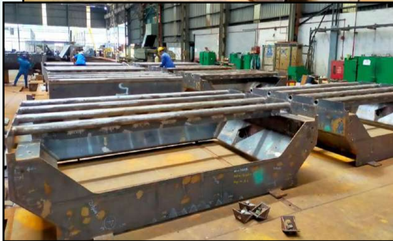
Fabrication of Grate Casing Tube
