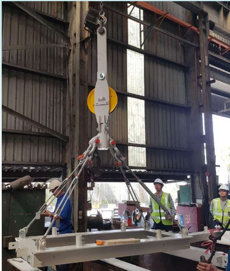
Temporary Hanging Scaffolding Setting
