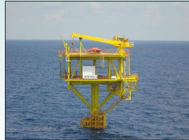
Bentara Topside site installation
