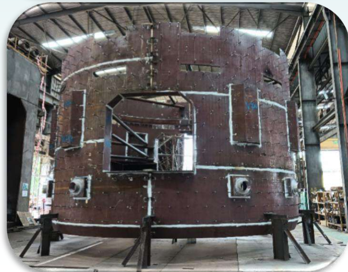
Pier Nose Liner
