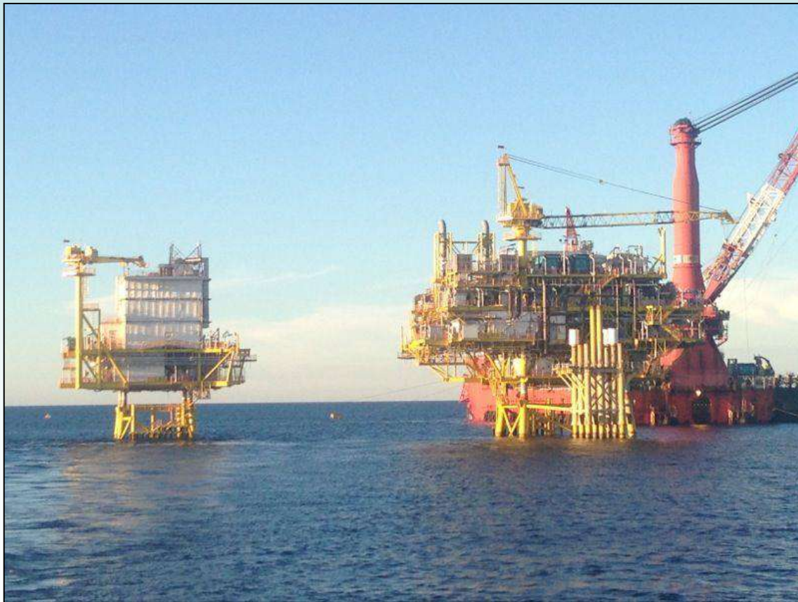
Living Quarter installed at site
