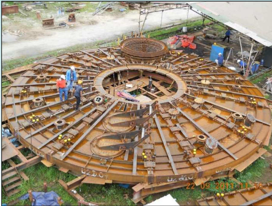
Water Cooled Roof Panels
